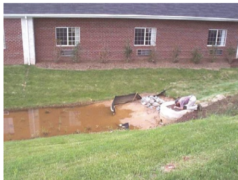
Bioretention area does not drain because of improper soil media, soils compacted during installation, and/or filter fabric under media.
