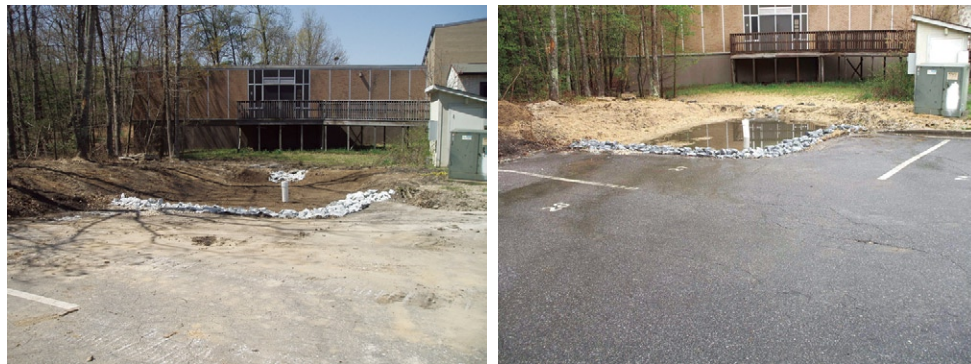
New BMP retrofit just after construction.
