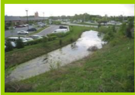
Failed infiltration basin to Wet Swale
