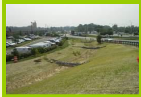
Failed infiltration basin to Wet Swale
