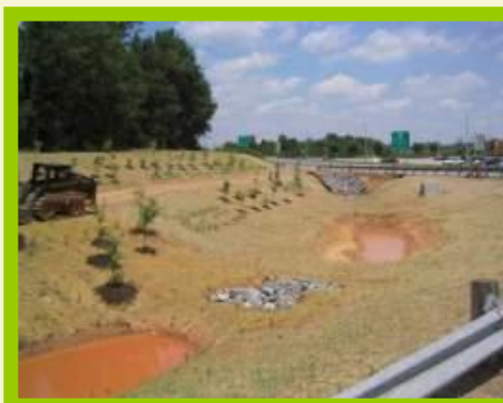
Failed infiltration basin to Extended Detention with Micro-pools
