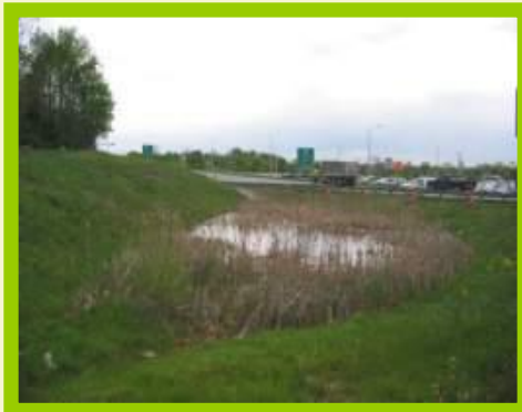
Failed infiltration basin to Extended Detention with Micro-pools
