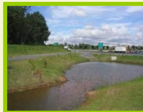
Failed infiltration basin to Extended Detention with Micro-pools
