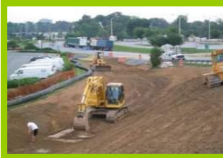
Failed infiltration basin to Wet Swale
