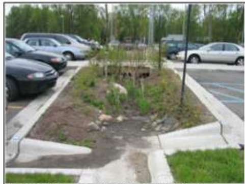
Bioretention area treating runoff from a parking lot
